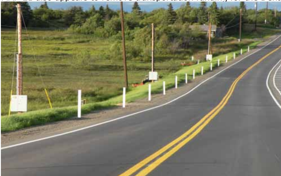
Dillingham's Wood River Road Project, 2010
