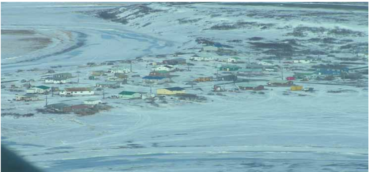
Aerial photo of roads in Twin Hills, Alaska
